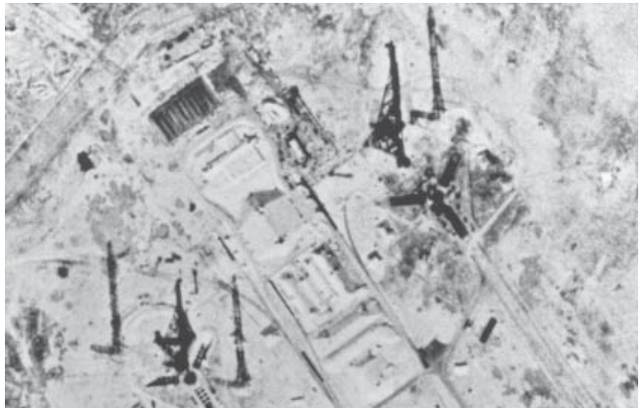
CORONA image of the launch complex after the devastating July 1969 explosion of an N-1 launch vehicle. (The large smudge on the right launch pad makes it clear that the vehicle exploded close to the ground. The flame trenches have been damaged and one of the two lightning towers around the pad has been destroyed.
