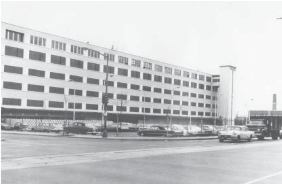
Building 213 in Washington DC which housed the secretive National Photographic Interpretation Center, or NPIC. NPIC was where all of the primary interpretation of satellite reconnaissance photographs was performed. Note that the windows on the first five floors have been bricked in for secrecy.
